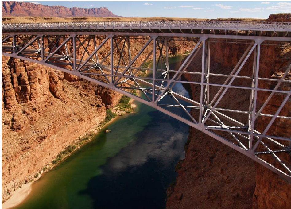
Colorado River at the Navajo Bridge
