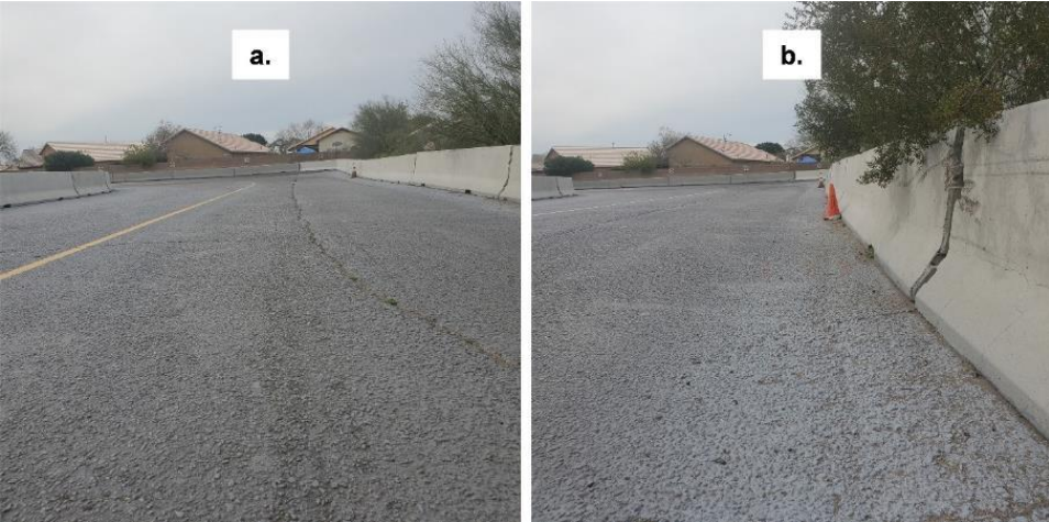
Figure 22. CP-A Section – March 2023; a. Wheel path; b. Shoulder.
