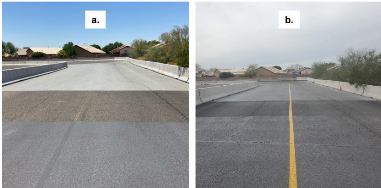
Figure 20 a. Test section in June 2022; b. Test section in March 2023.
