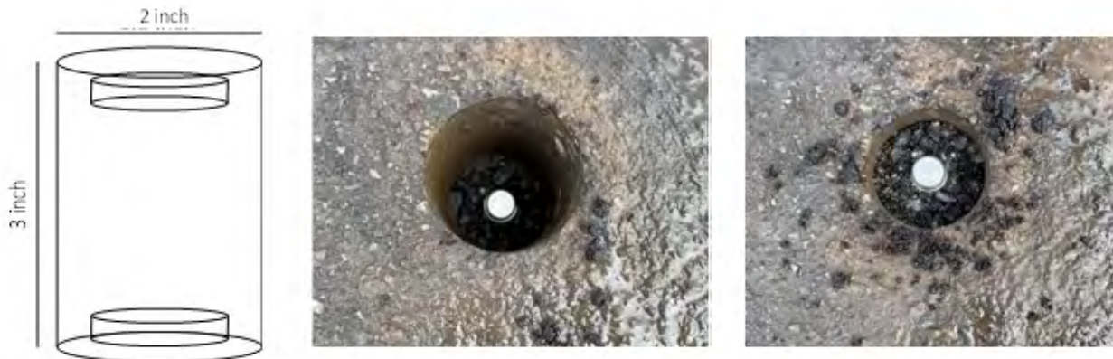
Figure 7: Temperature sensors (iButtons) are placed at ½ inch and 3 inches depth in the asphalt to measure subsurface temperatures.
