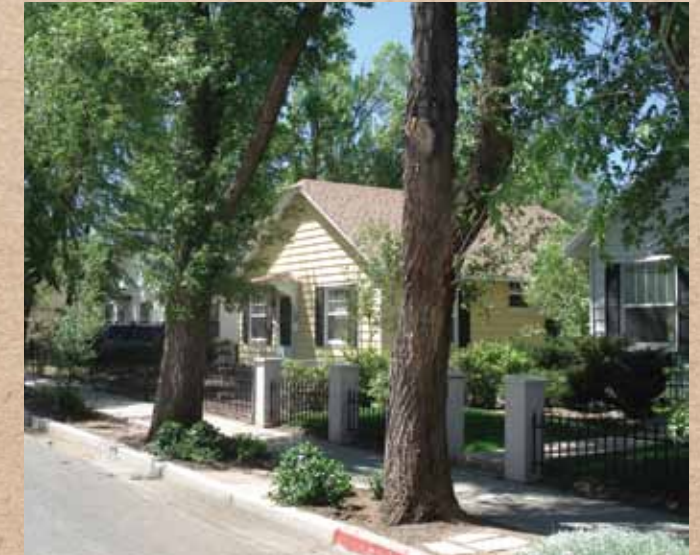
The City completed 31 rehabilitations in 2009 and 2010
