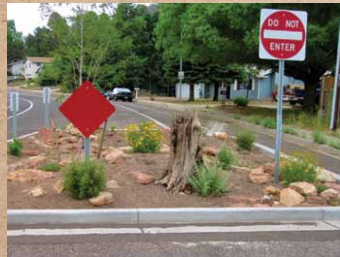
Stormwater irrigates the plants in this traffic calming device.
