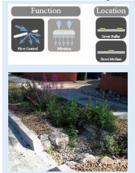
Figure 3 - LID toolkit example: curb cut for water harvesting
