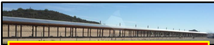
Solar canopy photo taken by researchers.
