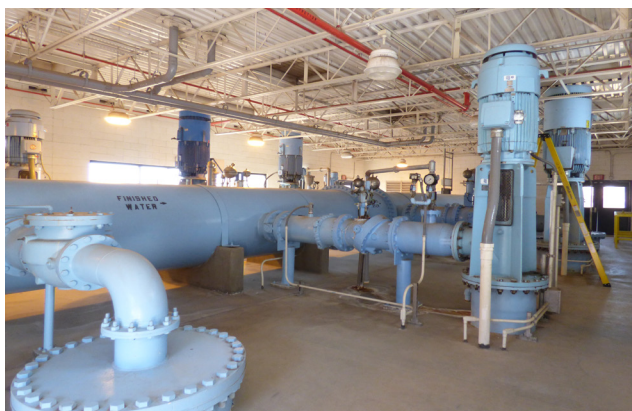
Figure 2a Water Treatment Facility in Peoria
