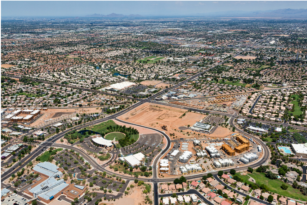
Figure 32 Gilbert, Arizona subdivisions and in-progress construction
