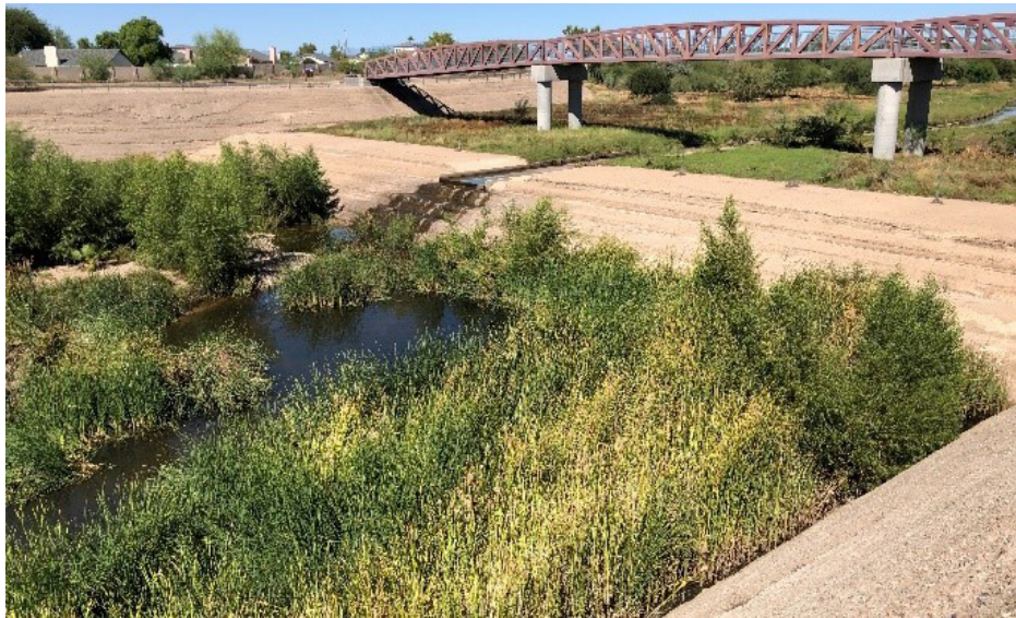
Figure 4 Typical water flows in the channel are minimal except during and after rain events, or monsoon season, as pictured here in early October 2019.
