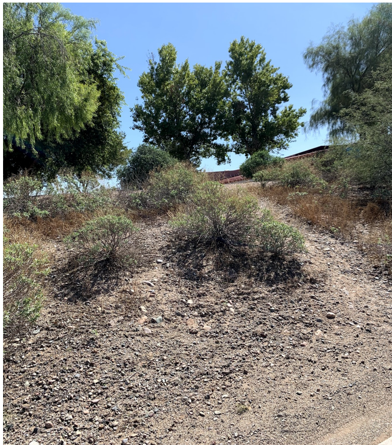
Figure 13 Embankment with a worn-in pedestrian path
