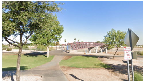
Figure 10 Existing pedestrian bridge near Rio Vista Recreation Center
