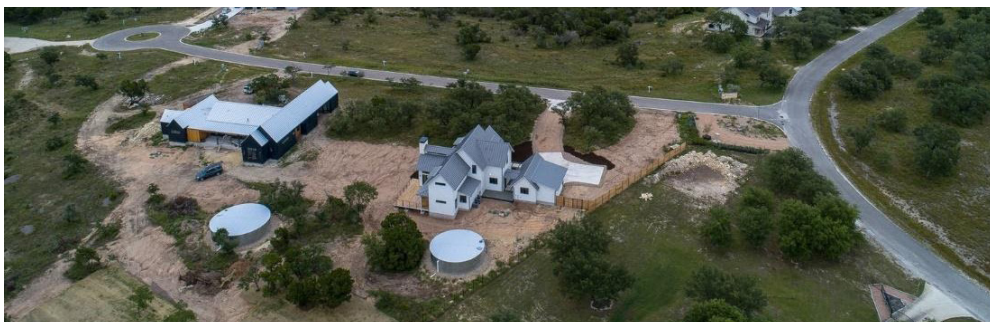
Figure 36 Aerial view of a property with rainwater harvesting and storage system, by Strong Roots Development
