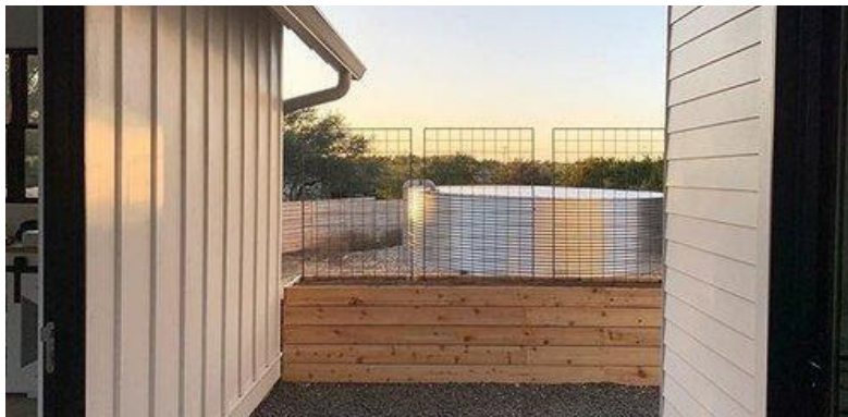
Figure 37 A Terra Scena home and its integrated rainwater harvesting equipment, by Strong Roots Development
