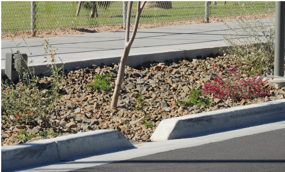
Figure 34 Curb cut and landscaped basin on Southern Avenue in Mesa's Fiesta District, by Arizona Water Facts
