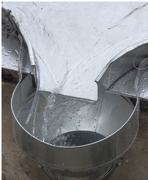
Figure 28 Rainwater flows into a catchment from a roof
