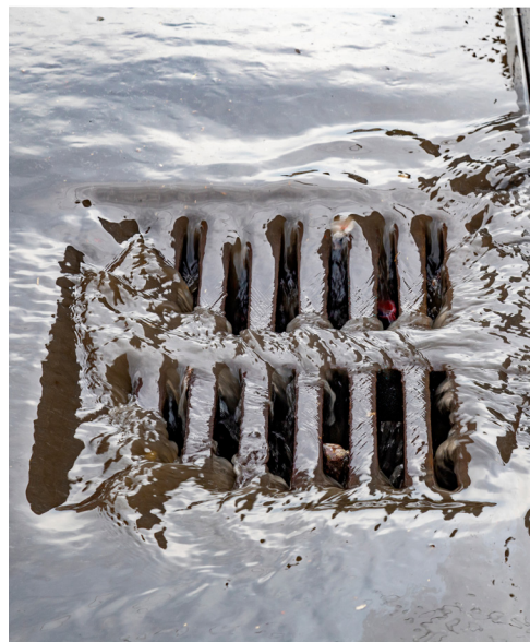
Figure 29 Stormwater flows into a street-level sewer
