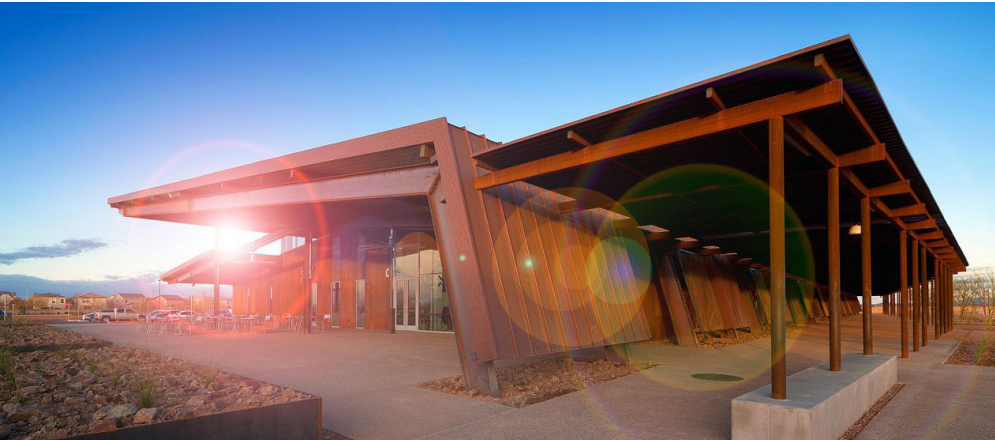
Clockwise from top left: CACZA hydrography of Apache Junction reveals water resources associated with 8,933.2 acres (p. 53); The amount of types of coverage in Apache Junction according to i-Tree (p. 55); Central Arizona College holds potential in the Economy & Jobs Goal Area (p. 39).
