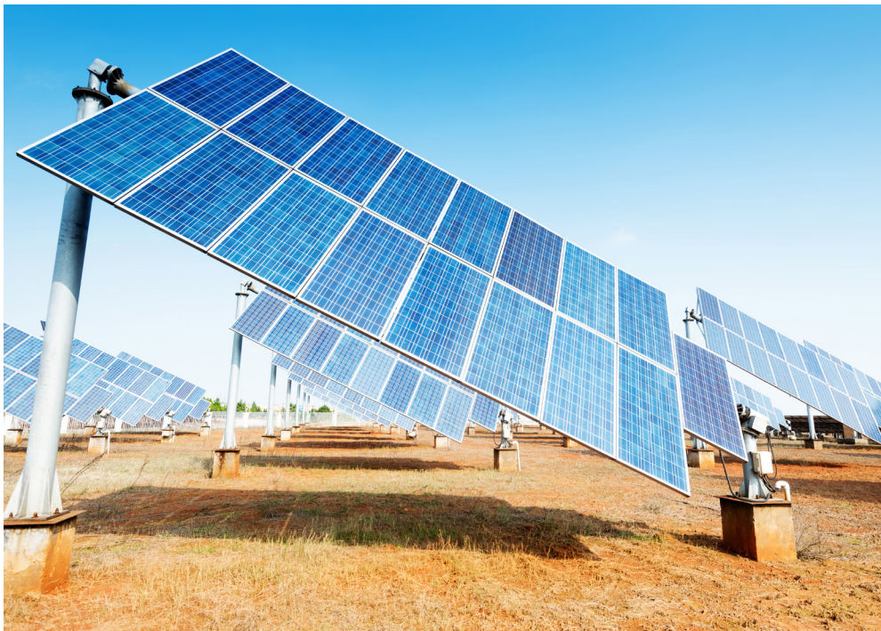
Figure 41 Example of a tracking solar panel setup, which tilts to maximize the amount of direct sunlight on the panel
