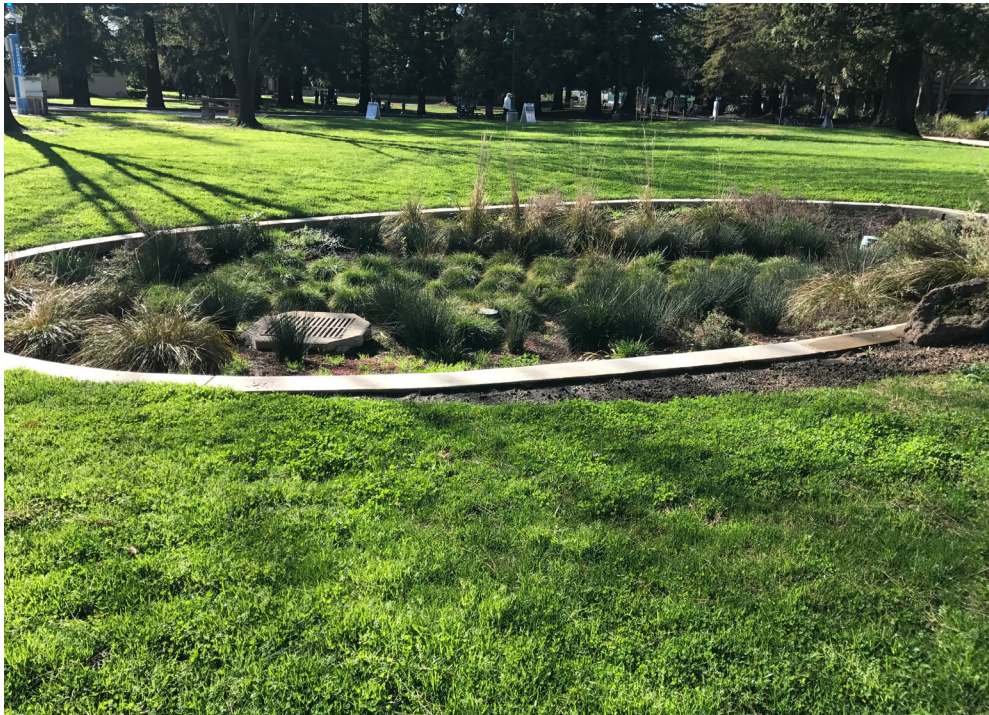
Figure 8 Rain garden which captures stormwater runoff to support native plant landscaping
