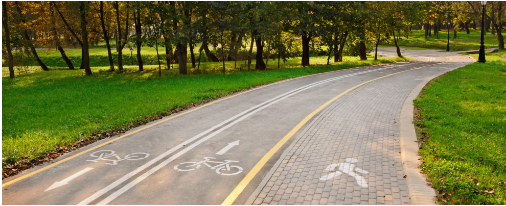
Figure 4 Example of a wide multi-use path, featuring designated bike and pedestrian lanes
