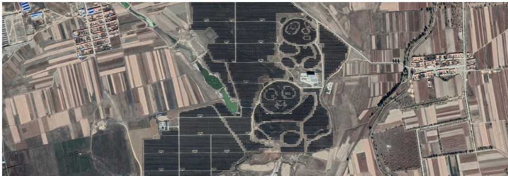
Figure 37 Panda bear solar array in Datong, China, via Google Earth
