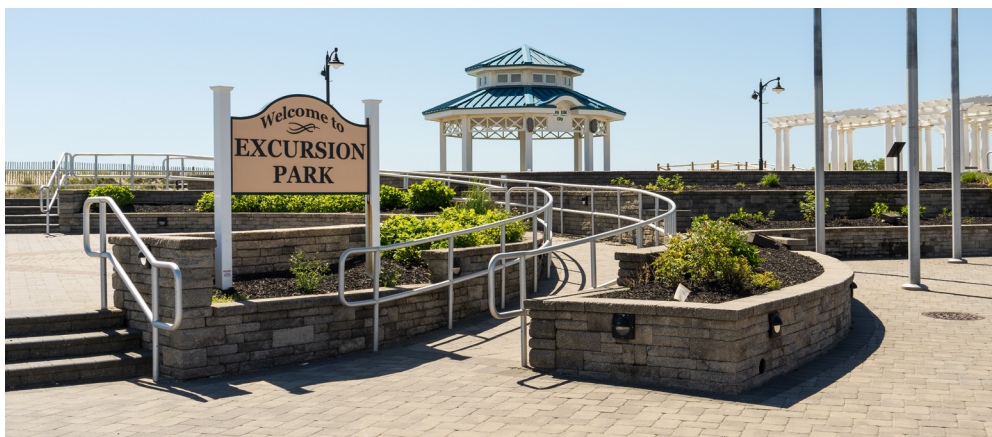
Figure 5 Example of an accessible ramp alongside stairs at the Excursion Park entrance in Sea Isle City, New Jersey
