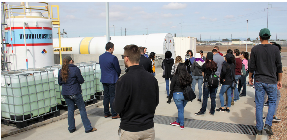
Figure 3 Students examine a number of Glendale's existing ASTs at the Oasis Water Treatment Plant
