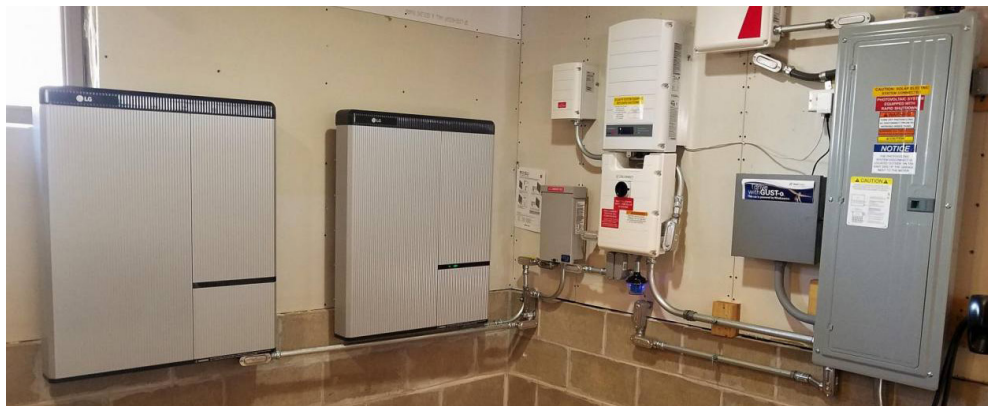
Figure 4 Installed residential solar battery system, by Brian Wolfson
