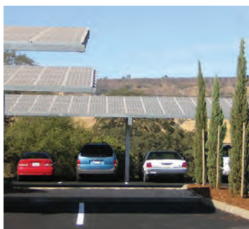
21B Solar panel shaded parking, by Great Valley Center via Flickr.
