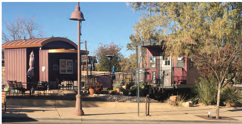
Figure 12 Clarkdale train car buildings on Main Street, by Neelam Shah.
