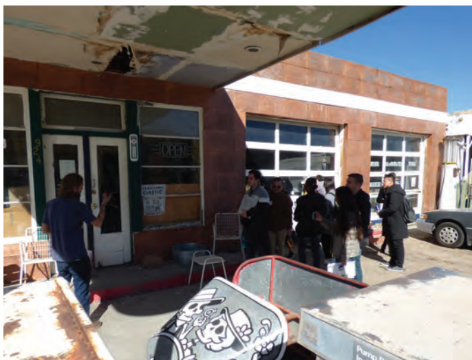
Figure 34 Clarkdale Classic Station owner opening the historic building for students to experience.
