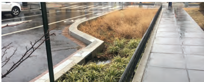
Figure 61 Bioswale separating a street from a sidewalk, by Eric Fisher via Flickr.
