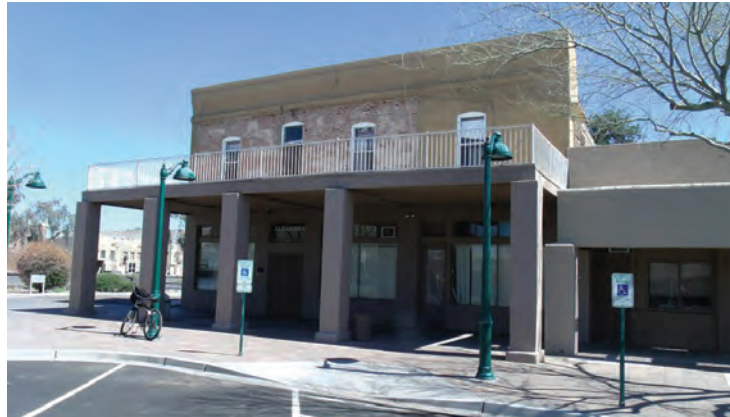
Figure 8 Downtown Mesa's historic Alhambra Hotel, which was redeveloped as student housing, via Wikimedia Commons.
