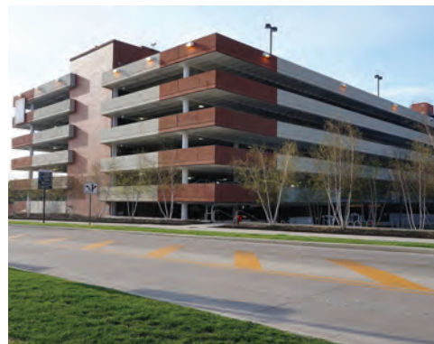
63B Large parking garage, by Maria Rimmel via Wikimedia Commons.
