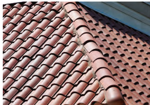
59B Clay tile roofing, by David Tribble via Wikimedia Commons.
