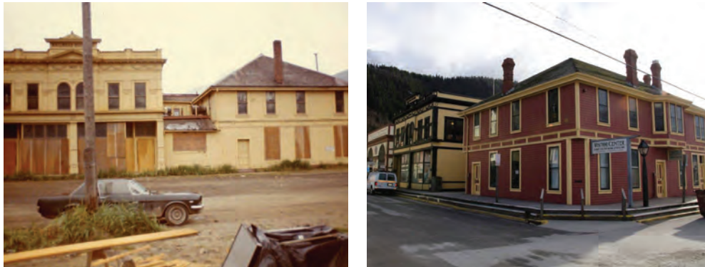
Figure 9 White Pass administrative and depot buildings in Skagway, Alaska, before and after rehabilitation with assistance from the National Historic Preservation Act. Retrieved from the National Parks Service.
