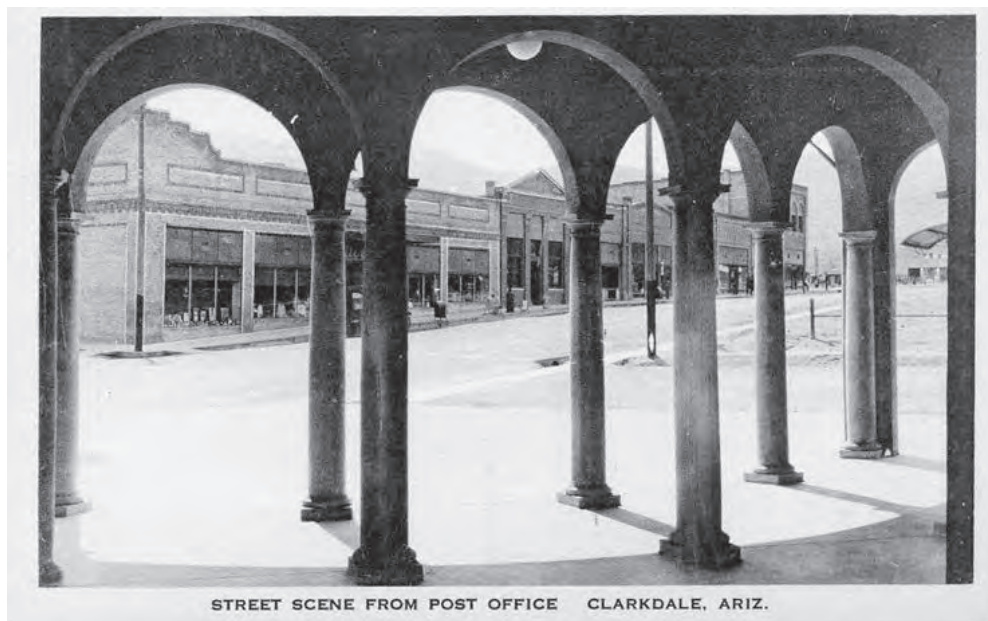
Figure 15 Clarkdale "Street Scene from the Post Office" postcard, by Town of Clarkdale.
