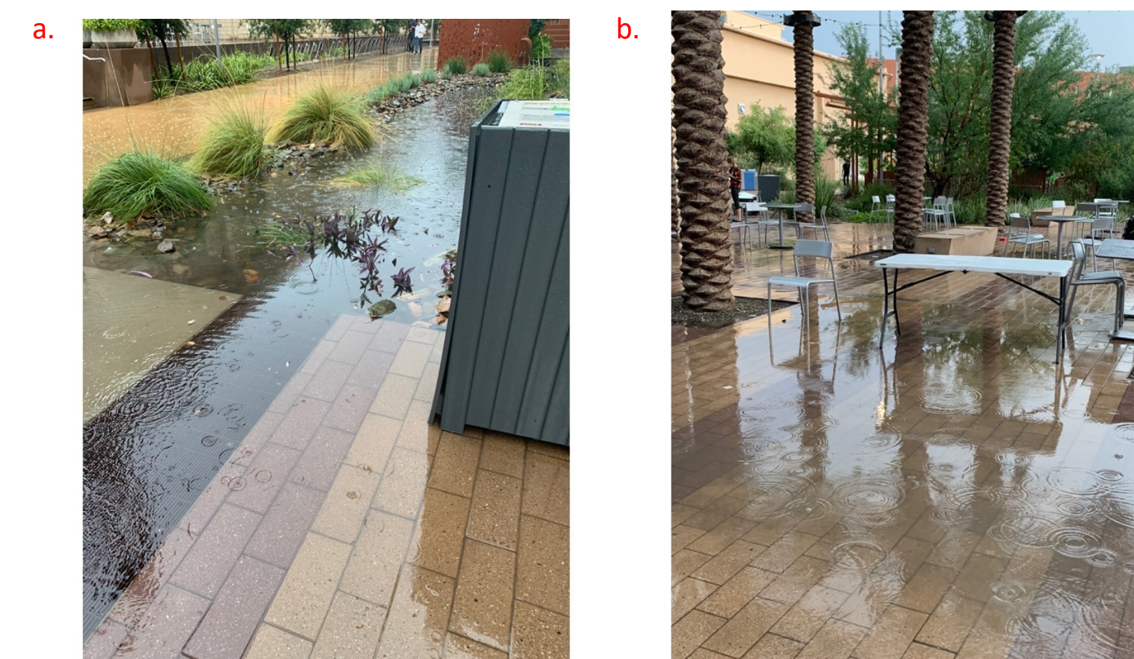
Fig. 6. a) Overflowing basin after heavy precipitation events from July 24-26, 2021. b) Example of water accumulating on impervious surfaces in Orange Mall.
