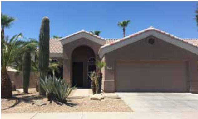
A typical newer home in Phoenix-area suburbs: built in 1995, xeric landscaping, a clay tile roof, and stucco walls.
