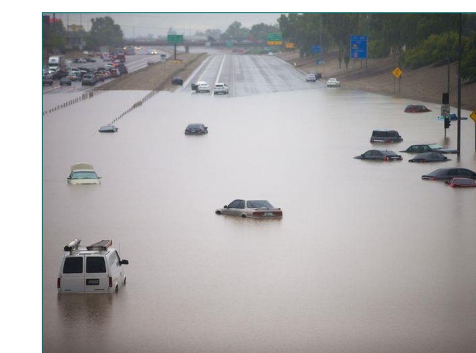
Image 2. I-10 failure in Phoenix, AZ (Michael Chow).
