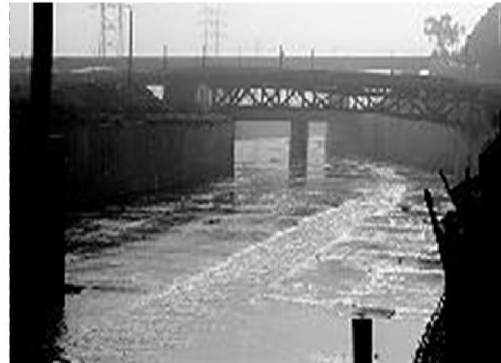
Figure 1. Storm runoff flowing down a canalized river channel. This runoff was created when rainwater landed within a common urban drainage basin (also referred to as a "catchment") and then gathered together along its downhill journey.
