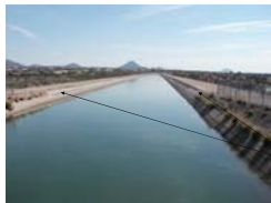
Figure 2: Due to subsidence and the resulting loss of freeboard, the canal liner (arrows) was raised at a cost of about $500,000 between Cactus Rd. and Shea Blvd. View from Cactus Rd. Bridge, looking downstream (southeast).
