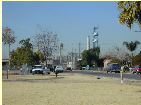
An APS power plant is located just west of Smith Park.
