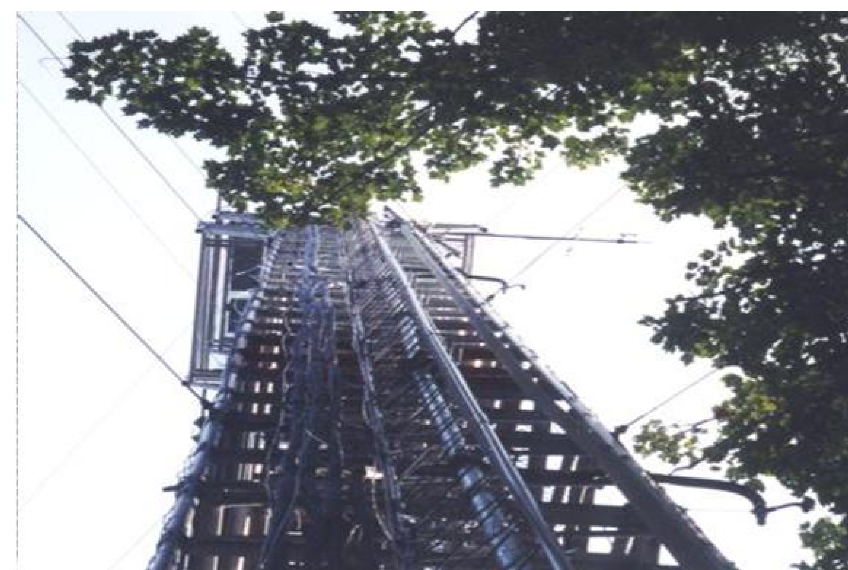
Figure 3: PROPHET tower at the University of Michigan Biological Station. Tower height is 31 m, forest canopy height is approx. 20 m.
